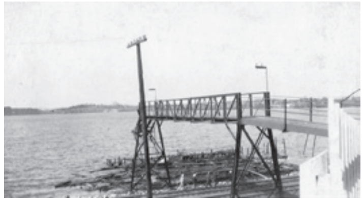
This is all that was left in the aftermath of the fire—only the metal bridge. Photo from the Scott Wheeler Collection
